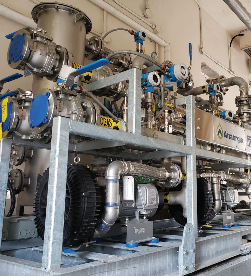
Biogas conditioning system installed at the Petawawa Water Pollution Control Plant in Ontario, Canada.
